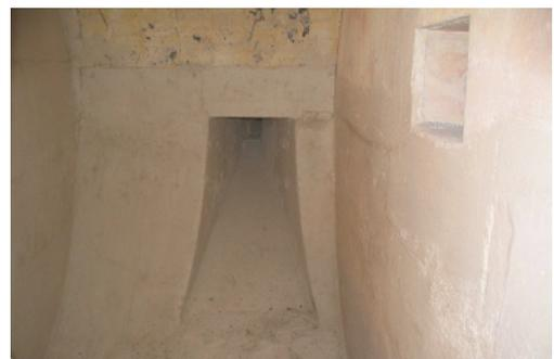
A tower melter lined with Capiral 85XS showing minimal deterioration after 12 months service.
